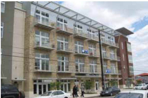
TwentyOne24 • East Austin Saltillo Plaza Station
