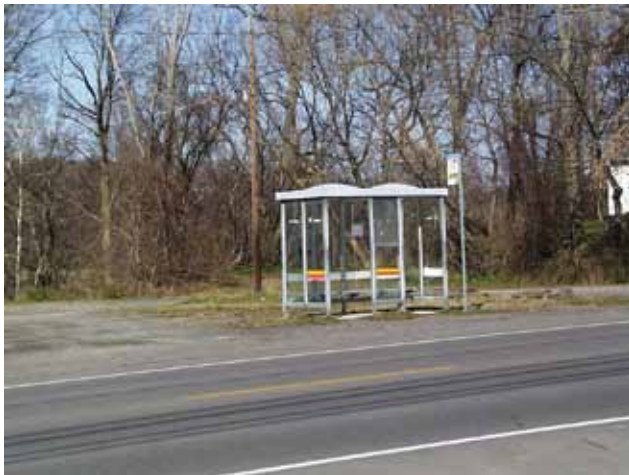
Example of bus stop without consideration of or complementing surrounding environment.
