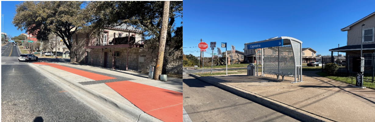
Pavement Rehabilitation and Bus Shelters
