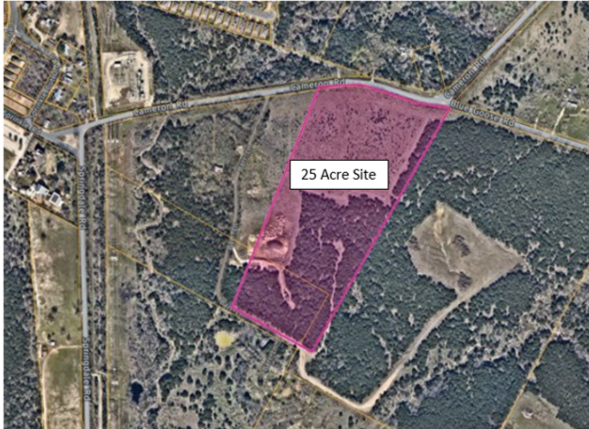
Site of North Base Demand Response Facility
