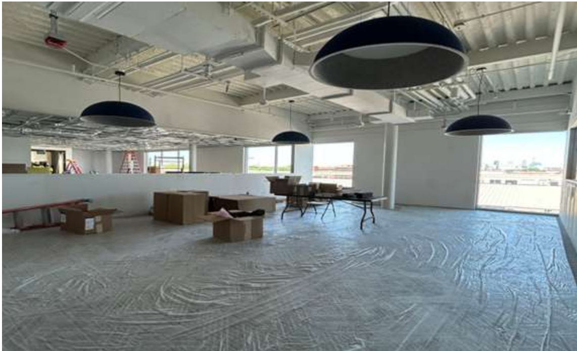
3100 East 5th Street Renovations
