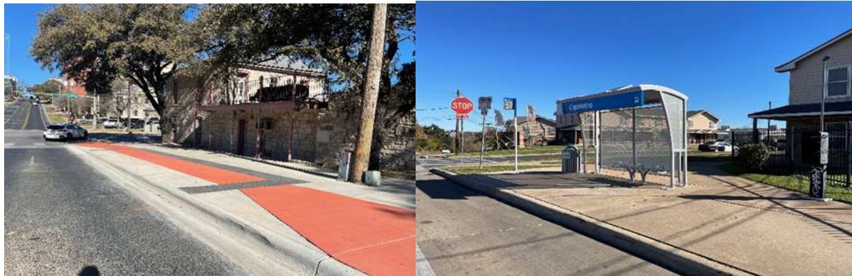
Pavement Rehabilitation and Bus Shelters
