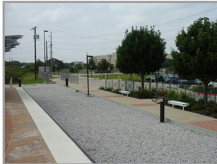
Research and development on Howard Lane opposite entry into Park & Ride
