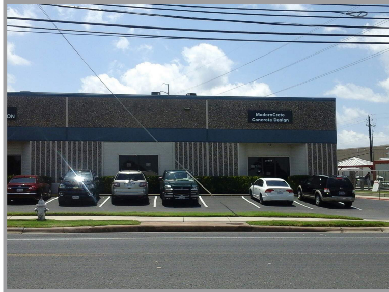
Warehouse/showroom lease space on east side of platform
