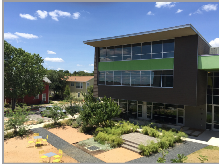
MLK Jr MetroRail Station is home to a variety of non-profit businesses and services, including PeopleFund, Chestnut Commons is pictured on the left
