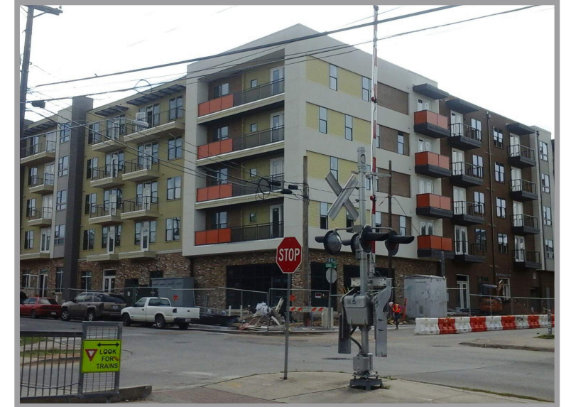
New, mixed use development surrounds the station area, this one on East 6th Street and Comal, The Arnold, includes offices, retail, and multi-family
