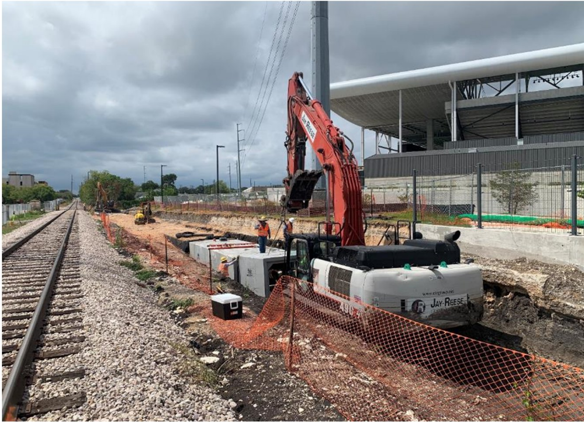
Main Culvert Install
