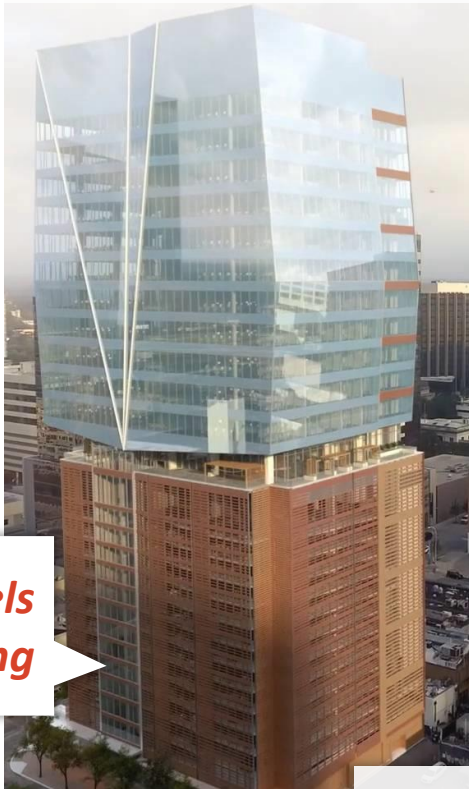
405 Colorado – breaking ground on 4 th and Colorado
