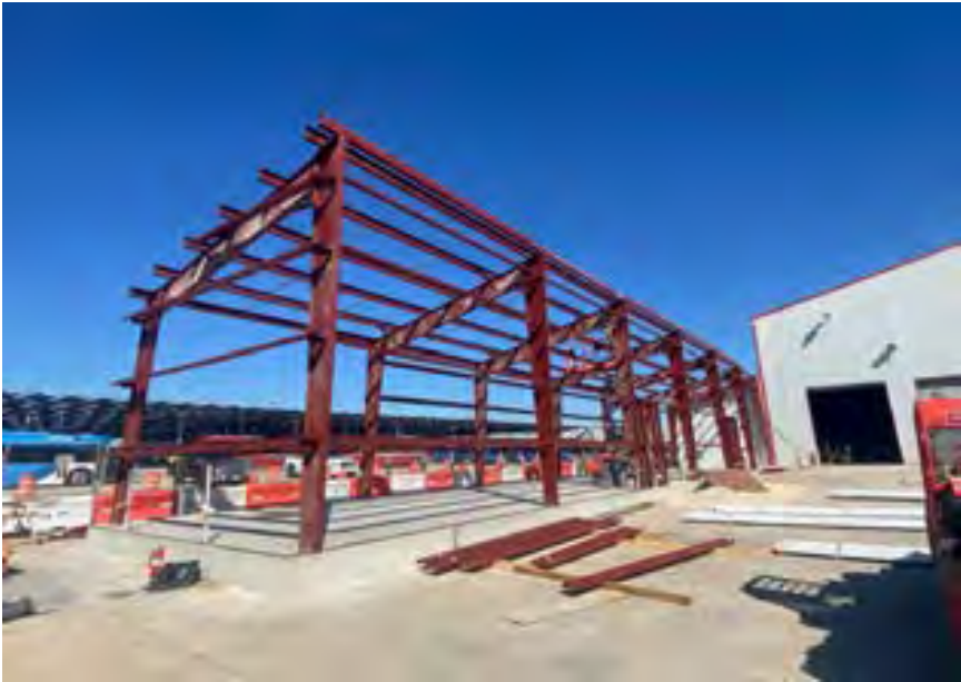
Steel Frame Erection
