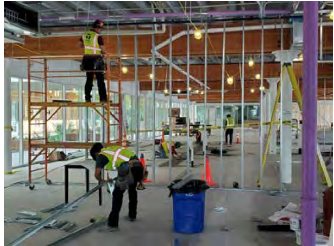
Wall framing at new Board Room lobby
