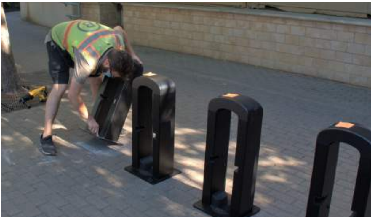
Figure 20: MetroBike 3.0 dock installation
